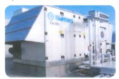
The FreeDry™ system uses the condenser side of a heat pump circuit to reactivate a desiccant dehumidification wheel. The efficiency of this cycle provides an extremely efficient reactivation input.
